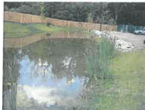
The retention basin at the CMHA Miles Pointe Senior Living apartments in Cleveland provides treats storm water and is a beautiful feature on the property.
